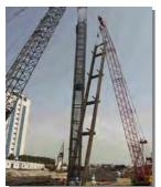
Lifting of O-cell assembly prior to installation
